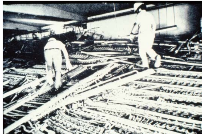
. Electro-mechanical equipment collapsed
