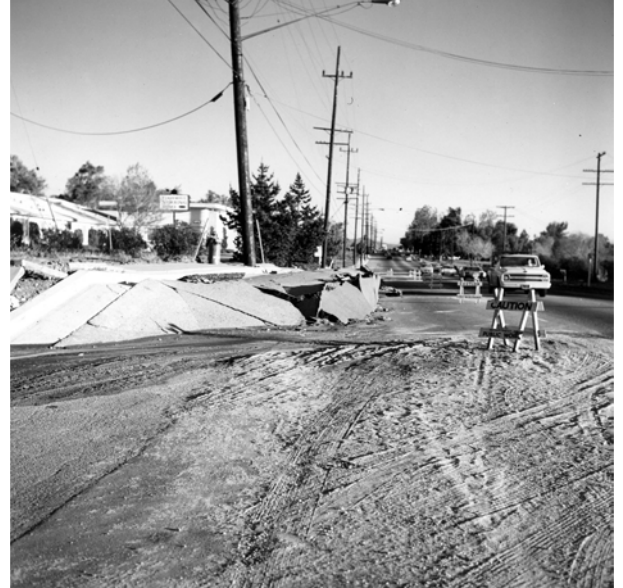
Scarp at Foothill Nursing Home – USGS Photo
