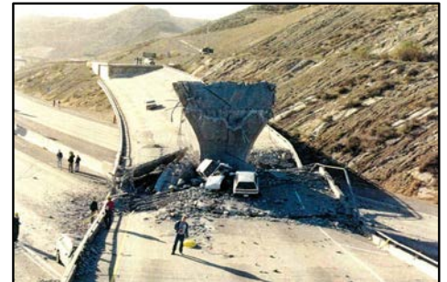
Route 14/5 Separation & Overhead
