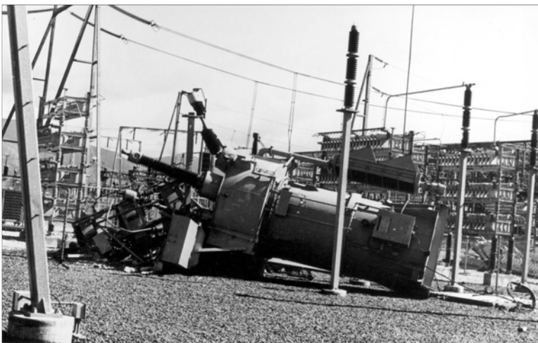
Damaged Power Equipment at Sylmar Switching Station – LADWP photos
