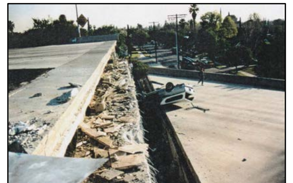
Mission Gothic Undercrossing
