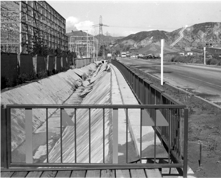
stormwater channel along Sepulveda Blvd. at Sylmar converter Station – USGS photo
