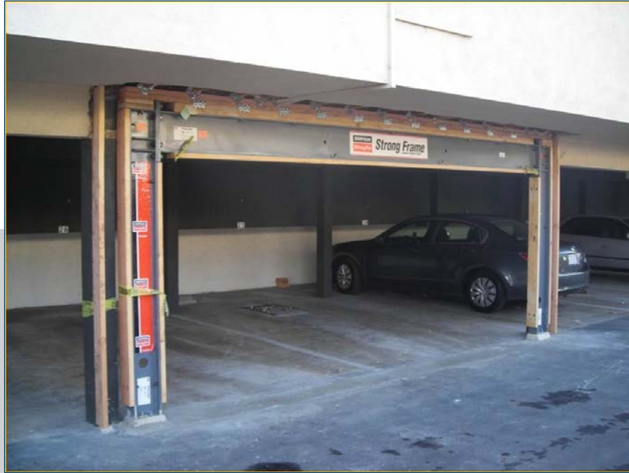
Steel frame around garage door opening
