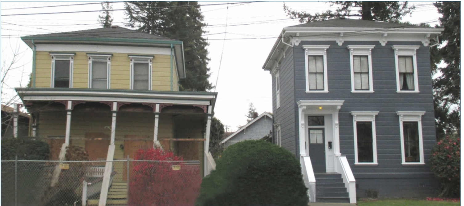
Unretrofitted - Red Tagged
