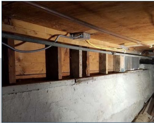
Crawlspace Before Retrofit
