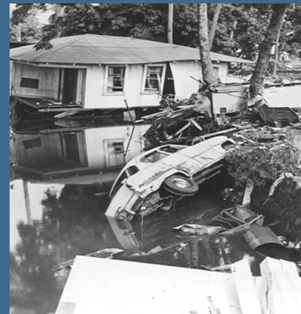
May 22, 1960, M9.5 Chile EQ Damage in Hilo, Hawaii
