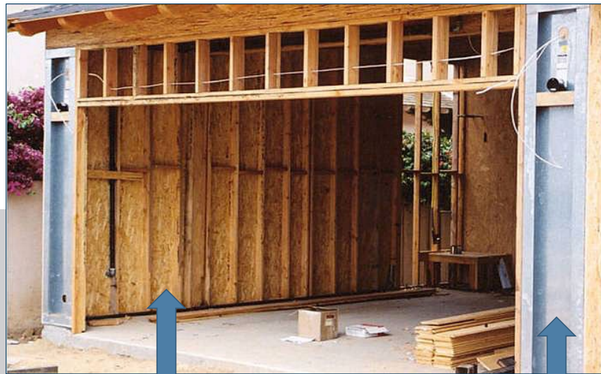
Plywood or OSB on first-floor walls
