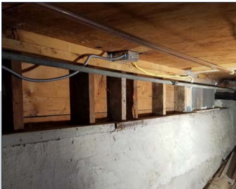
Crawlspace Before Retrofit
