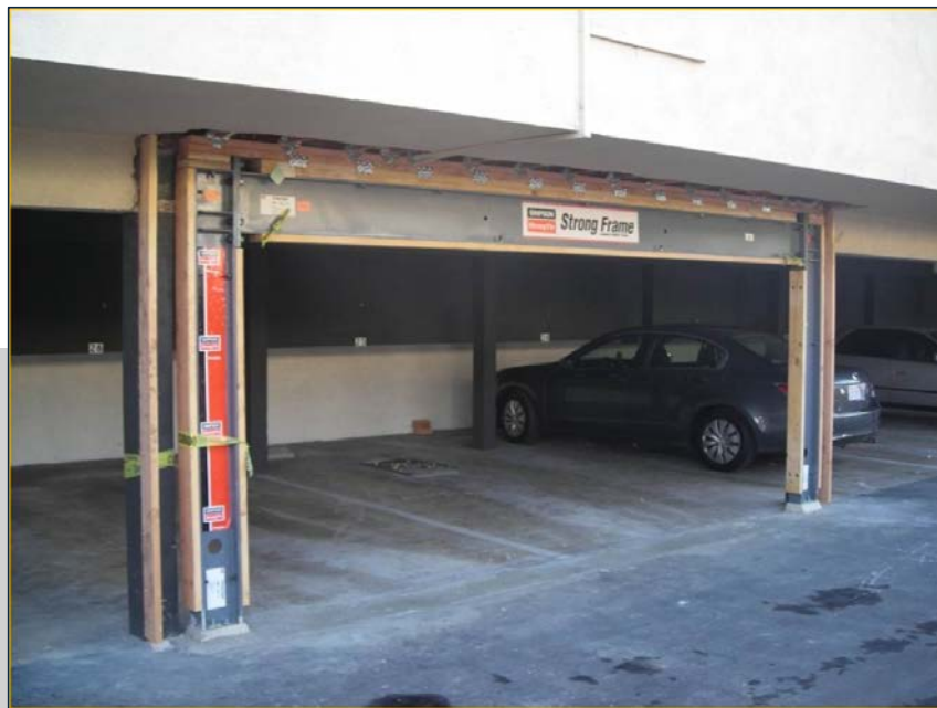
Steel frame around garage door opening
