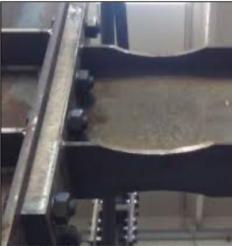
Fig. 1. Typical shape of a "Dog-Bone" connection
